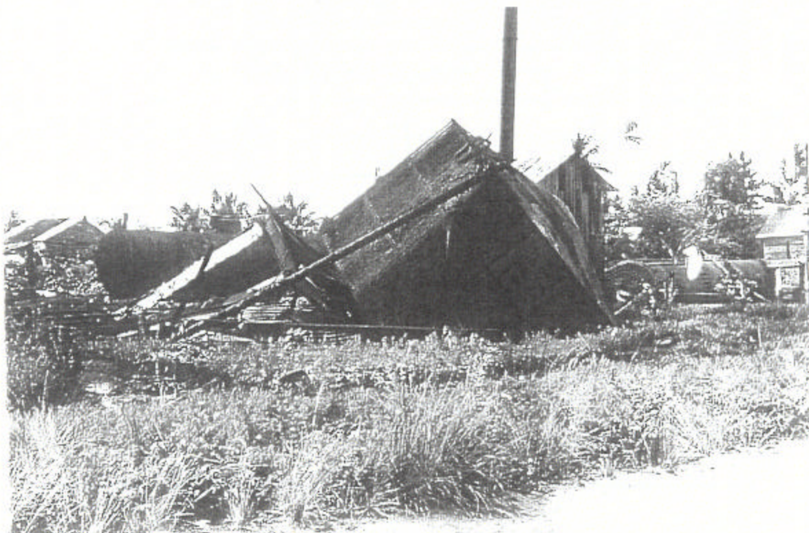
Photo 1. Reduc tion of the foun da tion bearing capacity and extru sion because of the seismic pore water pressure
