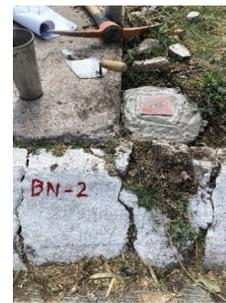
Figure 7. Final result of the placement of the GCP
