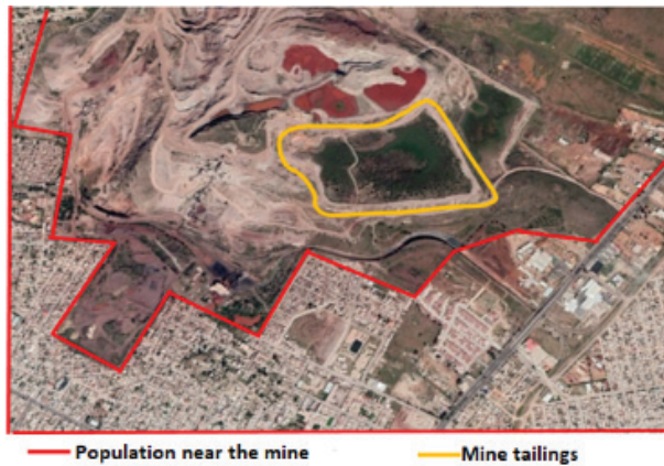
Figure 7. Population living nearby tailings dam
